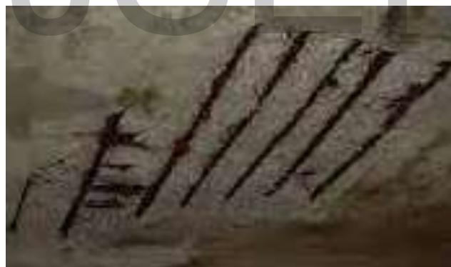
Fig. 1—Corrosion of steel bars.
